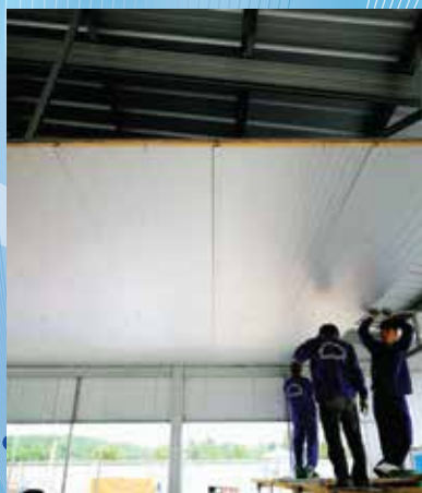
Flat PU Ceiling Installation
